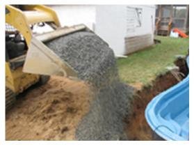
Once the plumbing is complete and the pool is set in the hole and leveled, it's time to start filling the pool with water and backfilling around the outside with gravel.
