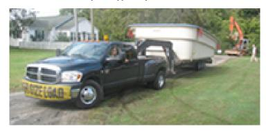
The pool will usually show up around lunch time of the first day, although it varies from job to job. Once the pool arrives, our team will unload it with the crane or excavator, set it on the ground, and begin installing the fittings and plumbing around the pool.
