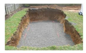
After the excavation is complete, we will place a 2–4" thick layer of gravel in the hole which the pool will rest on. This gravel base determines the height of the pool, so we use a laser level to set the gravel at precisely the right elevation. We are usually at this point at the end of day one or the beginning of day two of construction.
